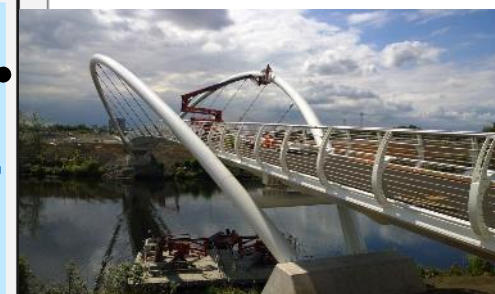
Dalmarnock Smart Bridge
